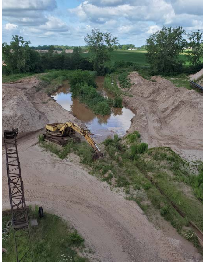
Looking west at sediment pond from top of plant
