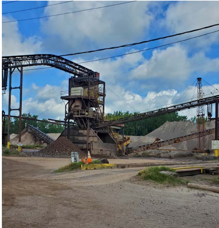
Looking northwest at plant from shop
